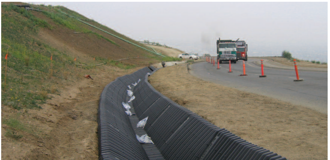
Initially, SmartDitch was installed in a channel at this Puente Hills Landfill site to temporarily control a conveyance ditch. However, considerable settlement over time made the use of concrete channels (originally specified) unusable and SmartDitch became the permanent solution.
