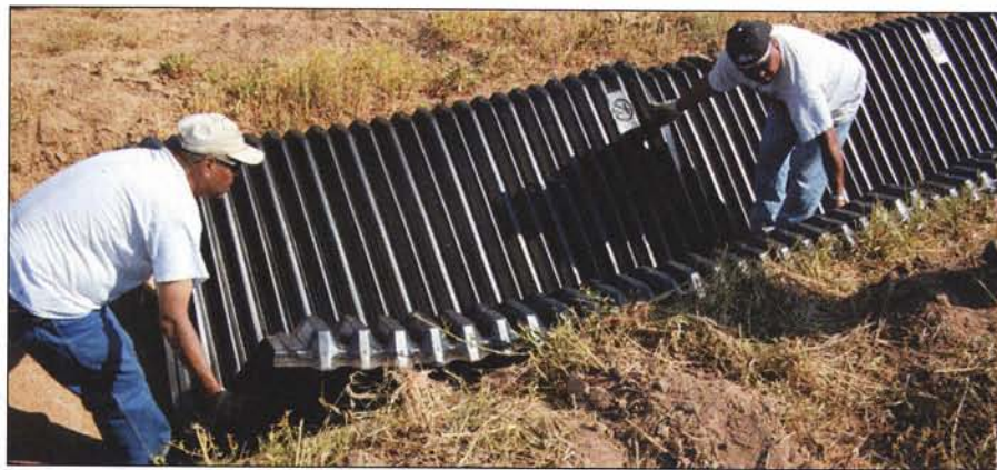
FLOW IMPROVEMENT: SmartDitch plastic liners recover lost efficiency from broken and decaying concrete ditches and canals.
