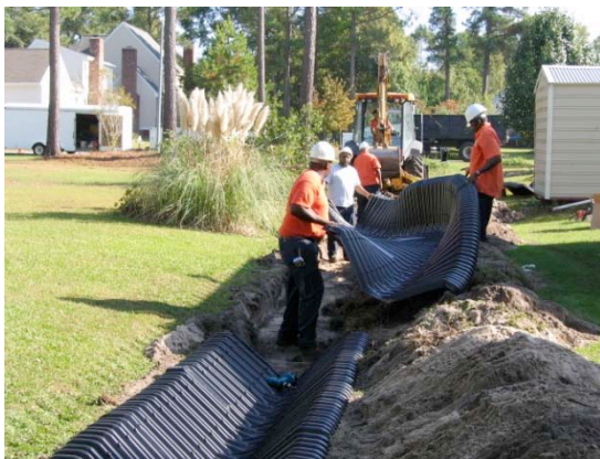
(City of Goldsboro Crews installing SmartDitch)
