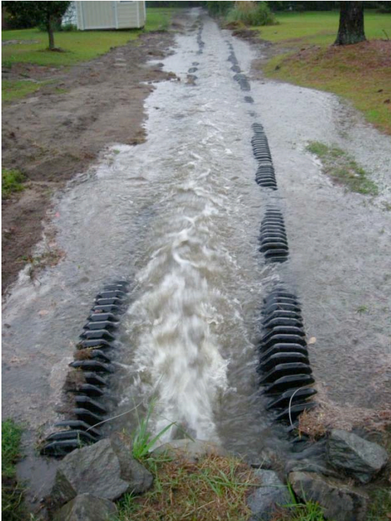
(Water flowing from a 15" Culvert pipe during heavy rain event)
