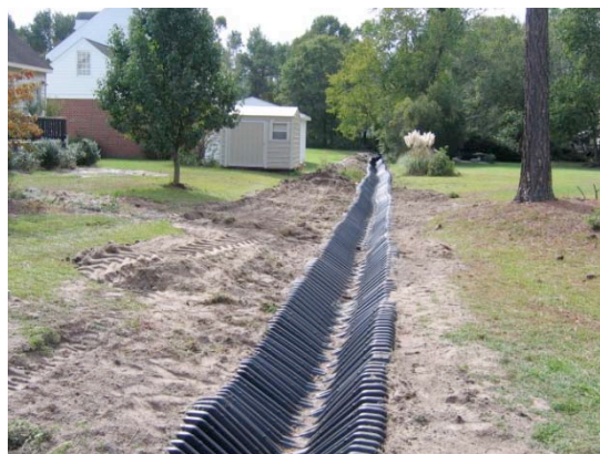
(320 lf of SmartDitch installed on first day)
