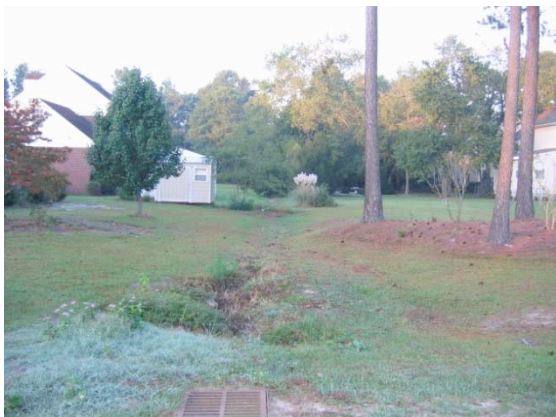
(Earthen ditch behind homes in Goldsboro, NC)
