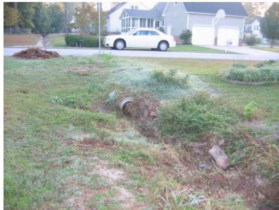
(The 15" culvert pipe that discharges into the ditch)
