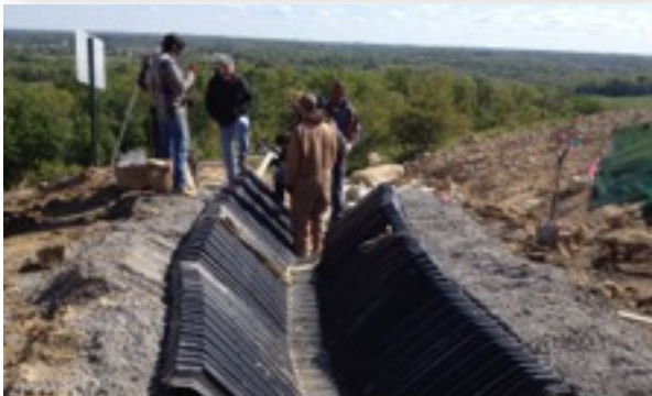
Installation took only two days to complete.
