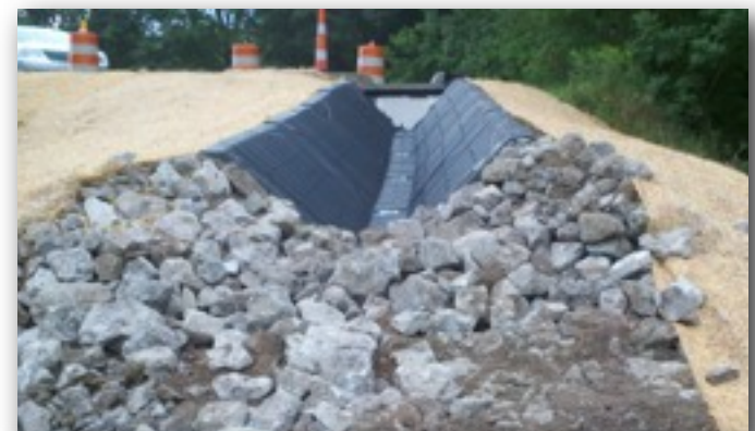
Completed spill with SmartDitch and repurposed rip rap
