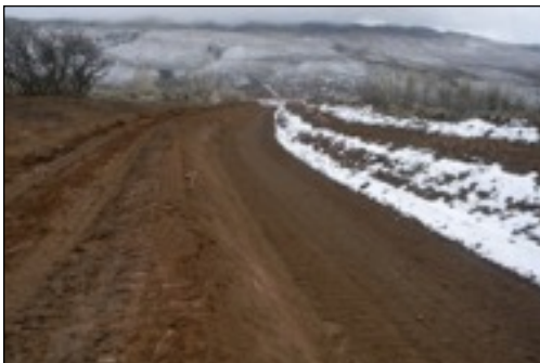
Soil conditions were perfect for a smooth installation.
