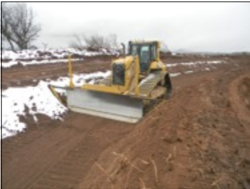
The contractor used a GPS guided blade to form the channel.
