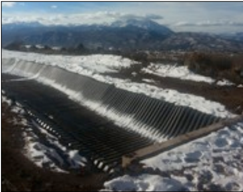
MegaDitch lined irrigation channel conveys much needed water to ranchers.
